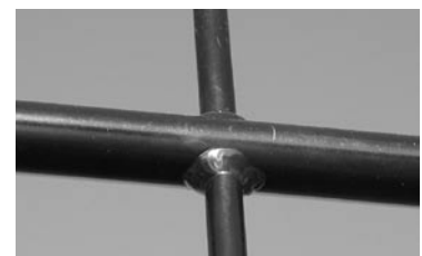
360° welded elements and black powder coating provide maximum durability
